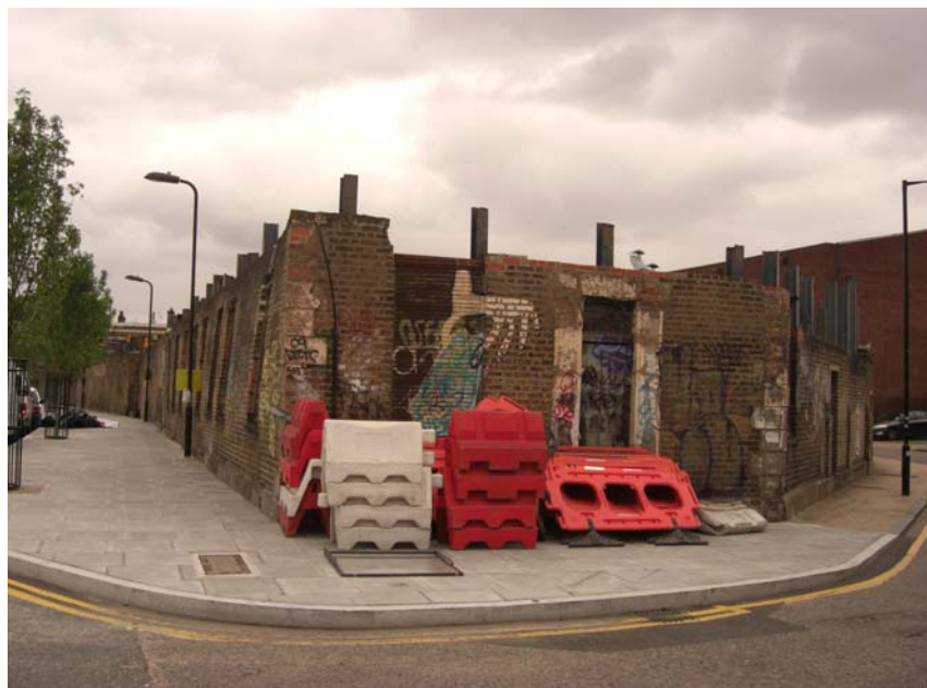
Figure 17 – Boundary wall on Wallis Road
