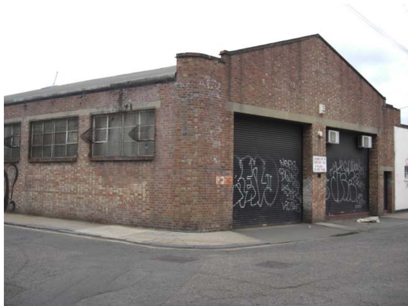
Figure 14 – No. 67 Rothbury Road/No.80 White Post Lane – circa 1953
