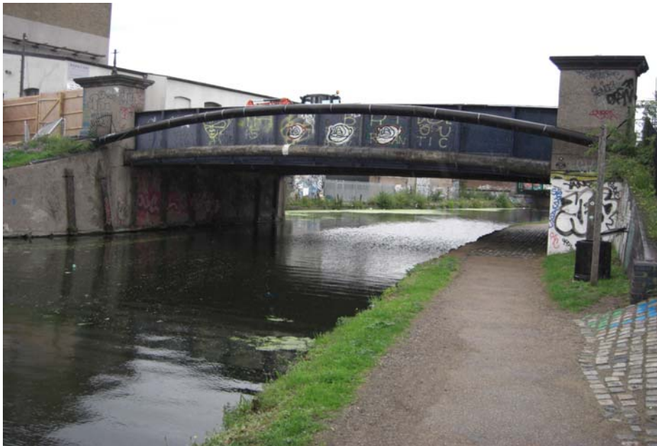
Figure 9 – Road bridge over the Hackney Cut – circa 1904
